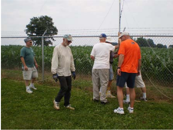
Antenna raising crew at work.
